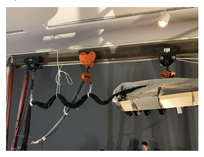
Have a person inside the sphere on a ladder that can come and receive the dome and make sure it fits within the brackets. Once it is in position, the person inside the sphere can insert screws loosely, and in the same fashion as for the other parts of the sphere, only tighten every screw once it is in place.
