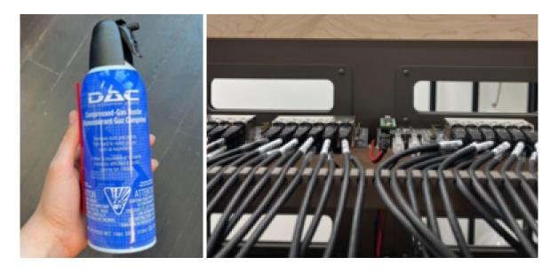
It is easier to reach the controller with the compressed-gas duster from behind like shown in the picture below.
