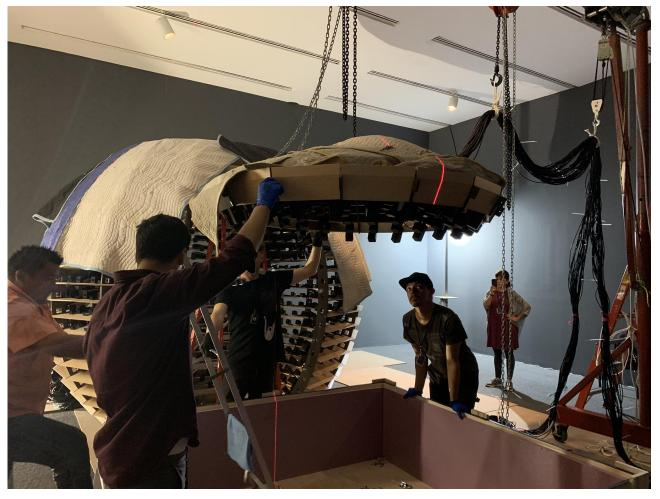
It is important to attach the cables onto the moving structure as well. They have a significant weight and it is important they do not "scrape" the side of the sphere (fragile wood slats).
