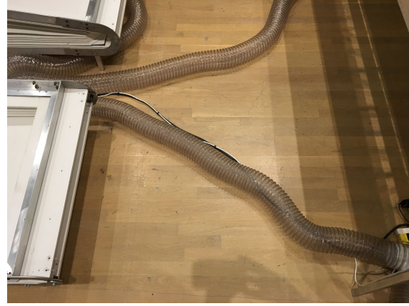
Power and data cables running under the hose to the valve table
