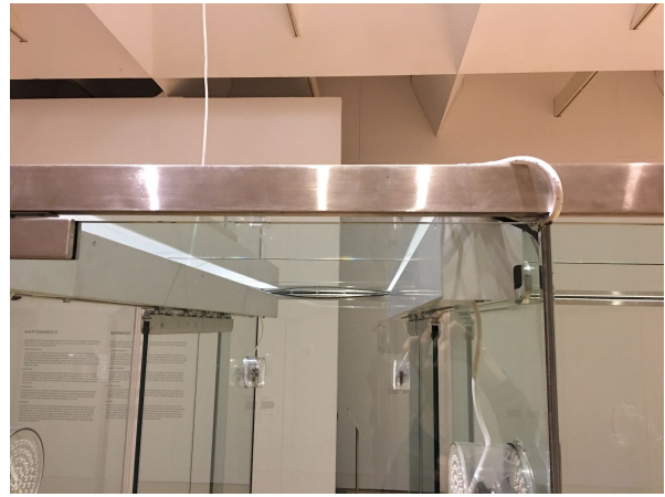
Power cable going to the inside of the second sliding door track. From there, it moves downwards, between the emergency doors
