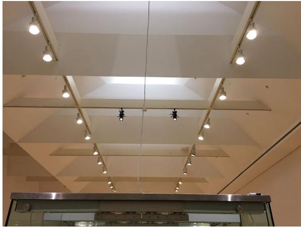
Power cable centered above glass chamber entrance
