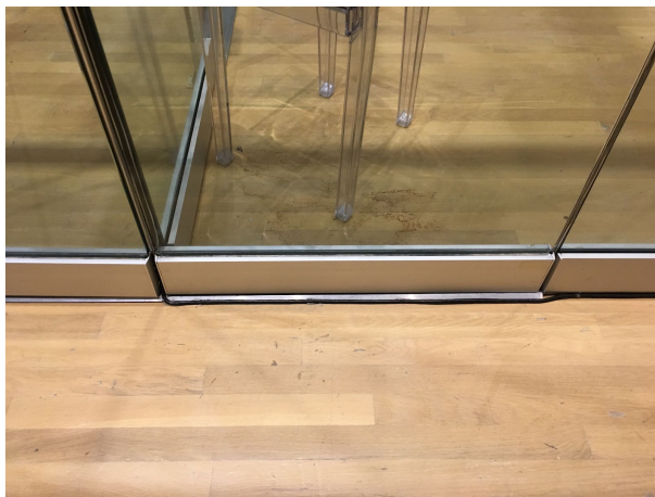
Black power cable running between the floor frame and the two emergency doors
