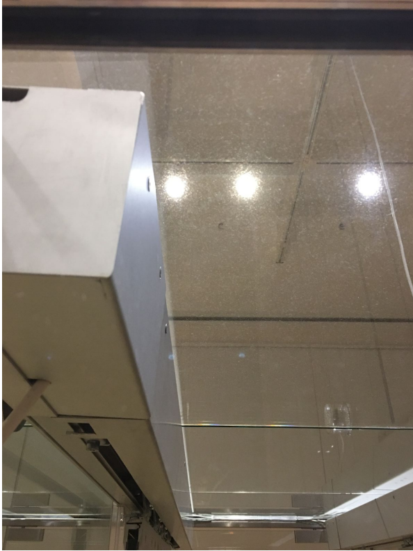
Dust on glass ceiling
